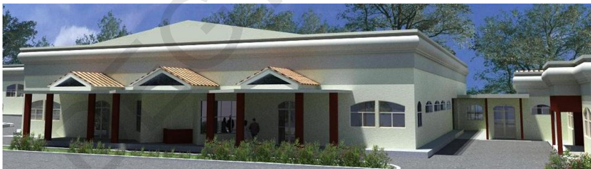
Figura No. 6 Fachada frontal del Hospital
